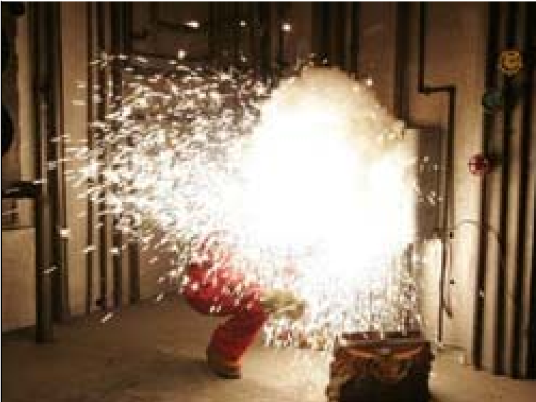
An arc flash blast can be deadly. A single phase-to-phase fault on a 480V system with 20,000 amps of fault current lasting for 10 cycles at 60 Hz will produce a blast equivalent to 1.5 lbs of TNT.
