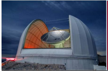
12 Meter Diameter; f/8 Observing season: October – June Carbon fiber construction Altitude over Azimuth Absolute pointing accuracy: 2.5" rms Tracking precision: 0.2" rms Efficiency: 85% +/- 5% Azimuth range: +/-270° Elevation range: 3° to 110° Observational range: ~18°- 84° Slew speed: 360° min<sup>-1</sup> Observational value: 60° min<sup>-1</sup> (Dome tracking limited) Supports position-switching, beamswitching, on-the-fly mapping, and continuum observing
